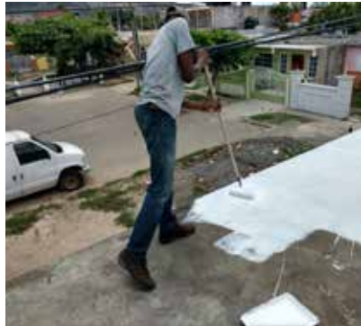
Fig. 4. Application of Sikalastic®-560 diluted with 10% water as a primer.
