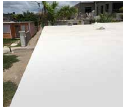
Fig. 5. Finished roof with 3 coats of Sikalastic®-560.
