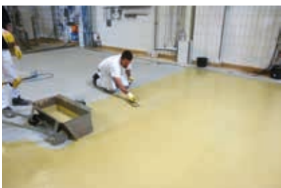
SATURDAY AFTERNOON: Application of the Sika® Ucrete® UD200 hybrid polyurethane flooring.
